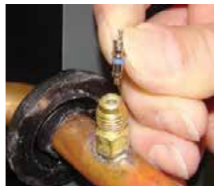
A. Remove the valve stem from the Schrader port mounted on the suction line.
