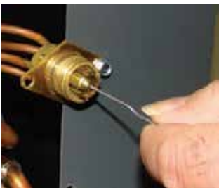
III-2. Remove the existing flowrator piston using a small wire or pick.
