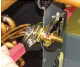
III-1. Disassemble the flowrator body using two wrenches. Unscrew the body with a counter-clockwise motion.
